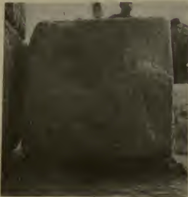
5. LEFT HAND END OF SLAB 4. SEE FIG. 3.
